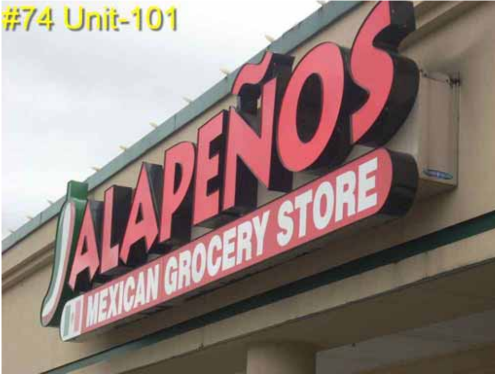
#75 Ceiling water stains
