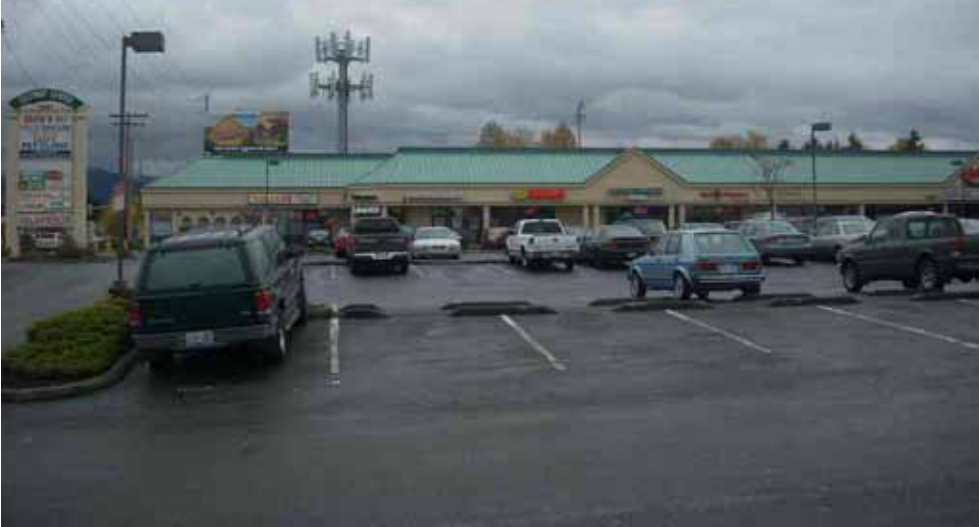
#4 -- 3901 West Wing and parking lot area.
